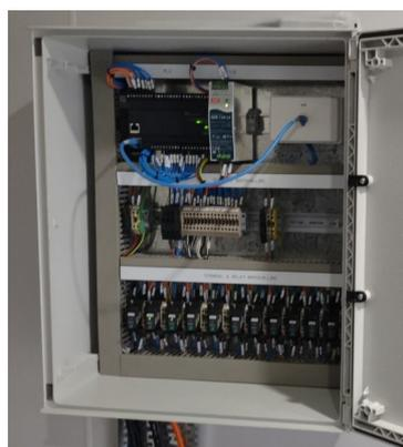
A PLC controls all of the field devices required for full weighbridge operation. This would usually consist of traffic lights, position sensors, alarms, etc.
